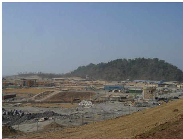
Oil and gas terminal in construction
