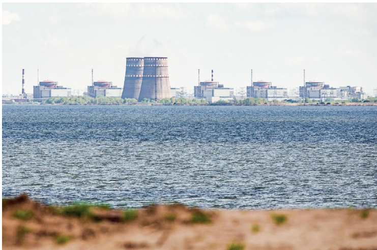
(FILES) In this file photo taken on 27 April 2022 shows a general view of the Zaporizhzhia nuclear power plant, situated in the Russian-controlled area of Enerhodar, seen from Nikopol. PHOTO: AFP
