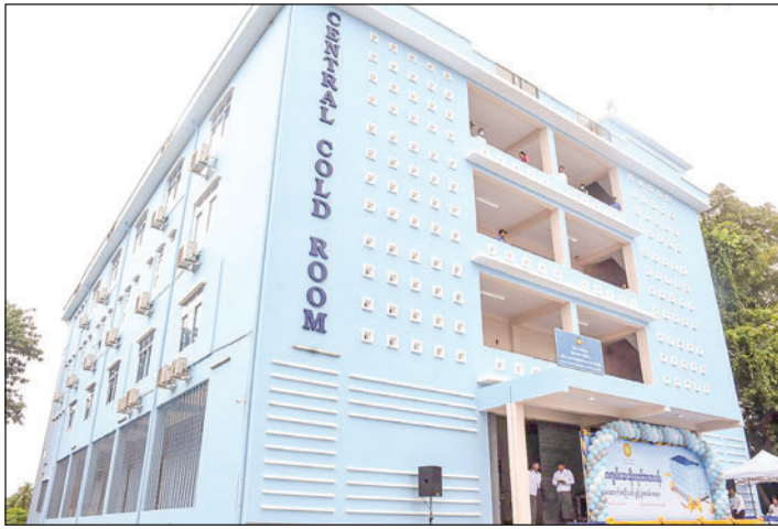
The four-storey central vaccine storage cold room (Yangon) in Mindhamma Road, Mayangon Township.
