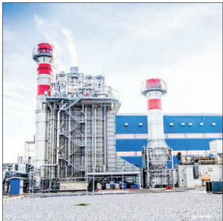
Myingyan power plant.
