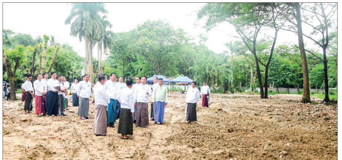
Union Minister for Information U Maung Maung Ohn inspects the Sarso Beikman construction site in Mingala Taungnyunt Township, Yangon, yesterday.
