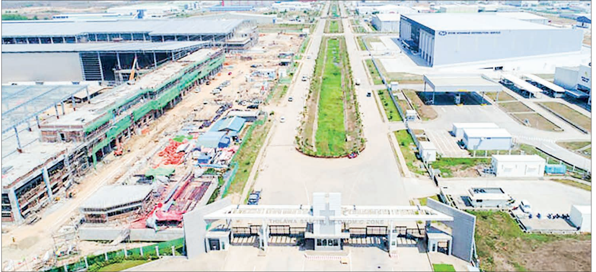
A panoramic aerial view of Zone B in the Thilawa Special Economic Zone in Thanlyan Township, Yangon Region. PHOTO: KANU
