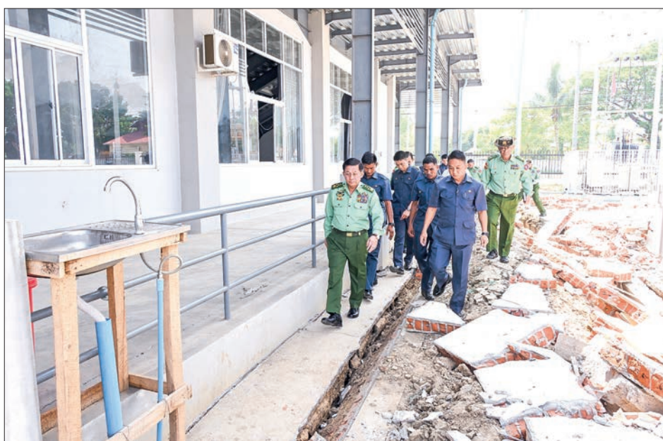
Inspection underway at the Nay Pyi Taw Stadium in Shwekyapin Ward.
