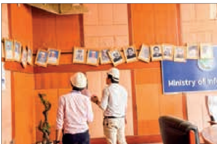
Construction experts conduct structural assessments of the Ministry of Information buildings following recent damage.
